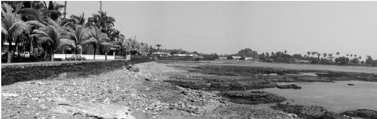
Figure 6. The seawall at the eastern end of Limón city and exposed coral raised by the earthquake of 1991 (Photo: Oscar Cuevas).
